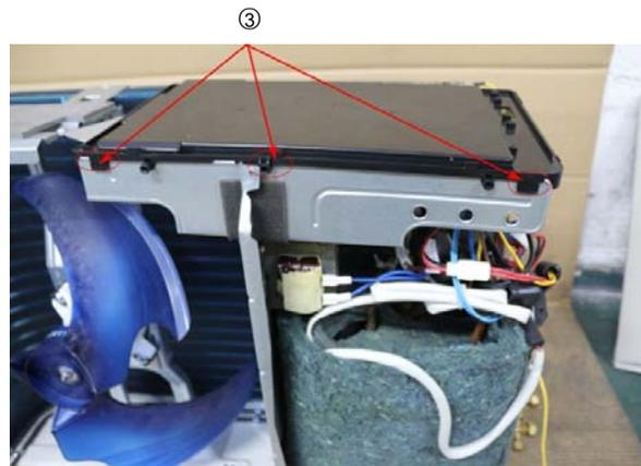
4) Disconnect the connector for fan motor from the electronic control board.
