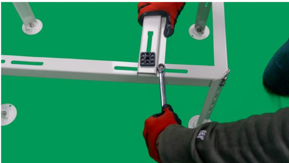
**Step 8: Measure and match the distance between the legs to that of the unit's mounting feet.**
